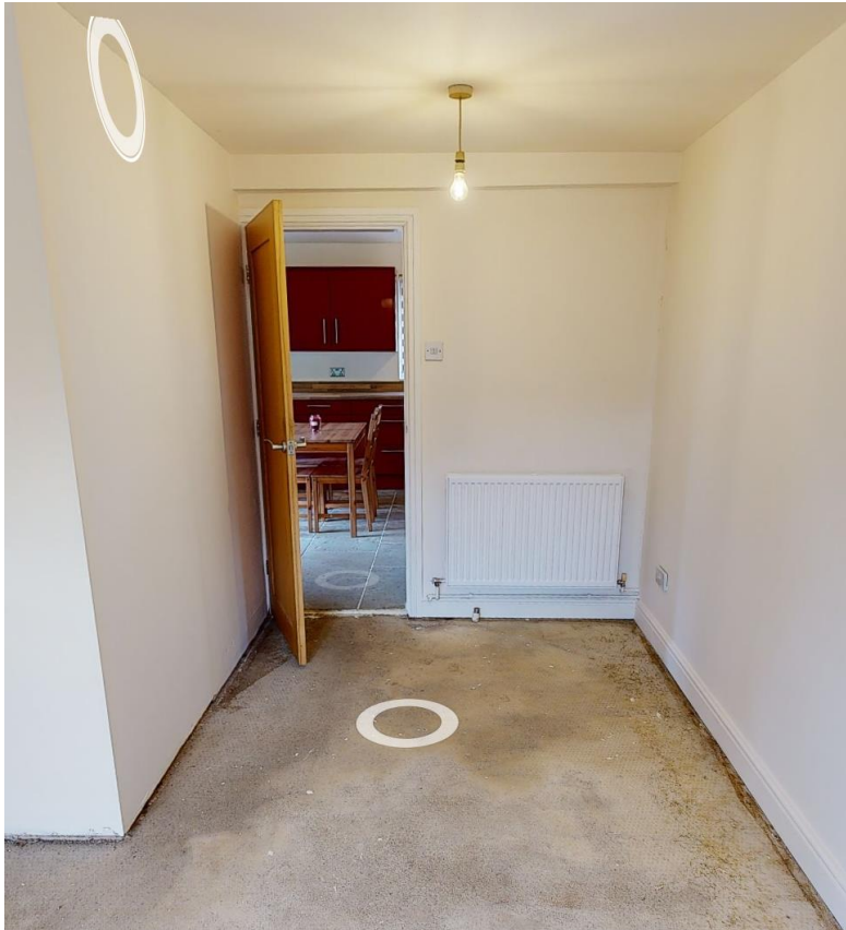
Figure 2: Image showing concrete screed in downstairs living area, and flagstones in kitchen, which are laid over original (1995) tiles.
